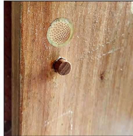
5. If wooden shafts and bearings expand, friction is created.
